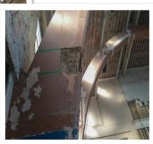
**The solution:** APA were contracted to design and install an impressed current cathodic protection system (ICCP) to masonry clad structural steel framed elements at Poplar Baths. Brick masonry was sympathetically removed to allow for the installation of the ICCP system
